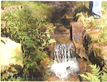
Water flow to be measured at Ridge SFH
