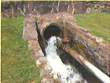
Water supply line at Petersburg SFH
