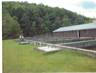
Reeds Creek SFH
