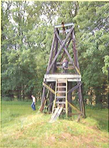
Water is pumped from the Little Kanawha River at Palestine SFH
