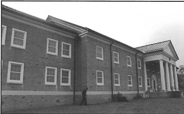
Division of Juvenile Services Jones Building Renovations Industrial, WV
