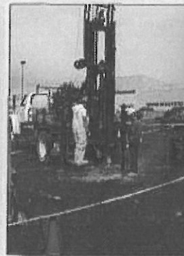
Drilling on Flat Terrain
