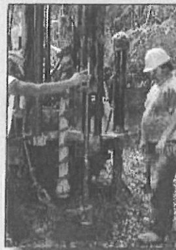
Drilling in Rugged Terrain
