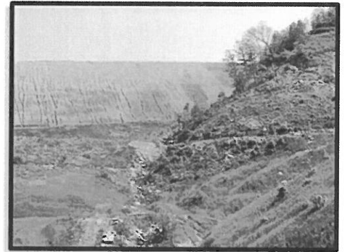
Downstream - Post Stage III Construction
