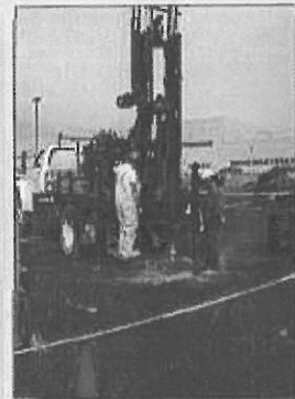
Drilling on Flat Terrain
