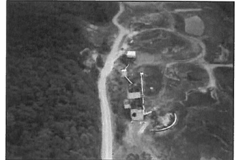
Site before Remediation
