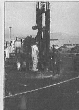
Drilling on Flat Terrain
