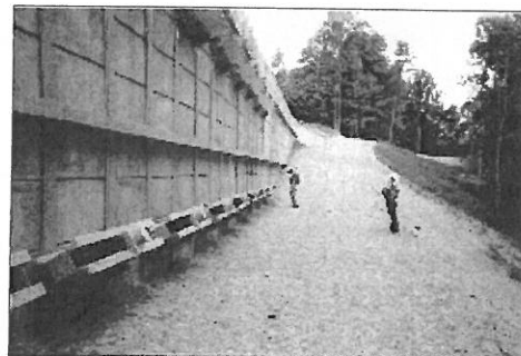
Finished wall with anchors
