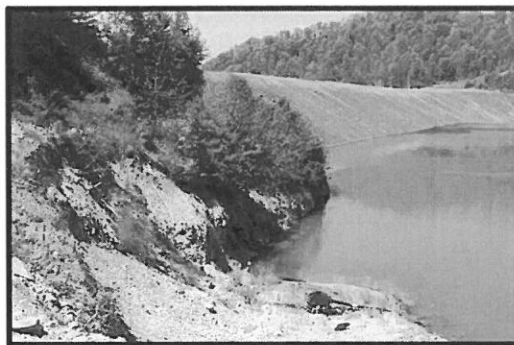
Upstream - Post Stage III Construction
