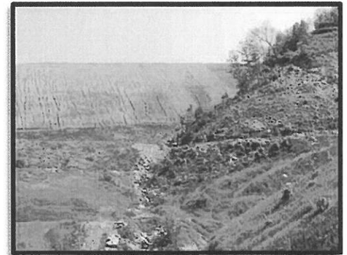
Downstream - Post Stage III Construction
