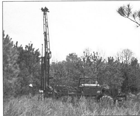
CTL's ATV can drill in rough terrain
