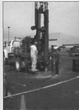
Drilling on Flat Terrain
