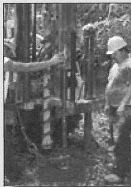
Drilling in Rugged Terrain
