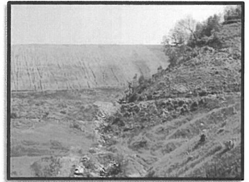
Downstream - Post Stage III Construction
