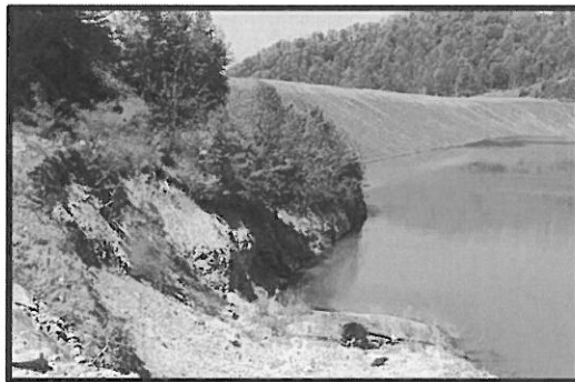
Upstream - Post Stage III Construction
