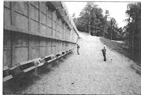
Finished wall with anchors
