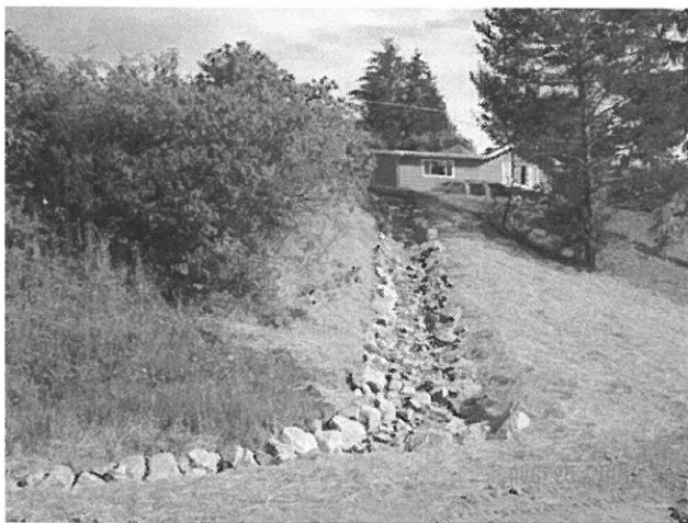
Erosion Repair – Rip Rap Armored Ditch
