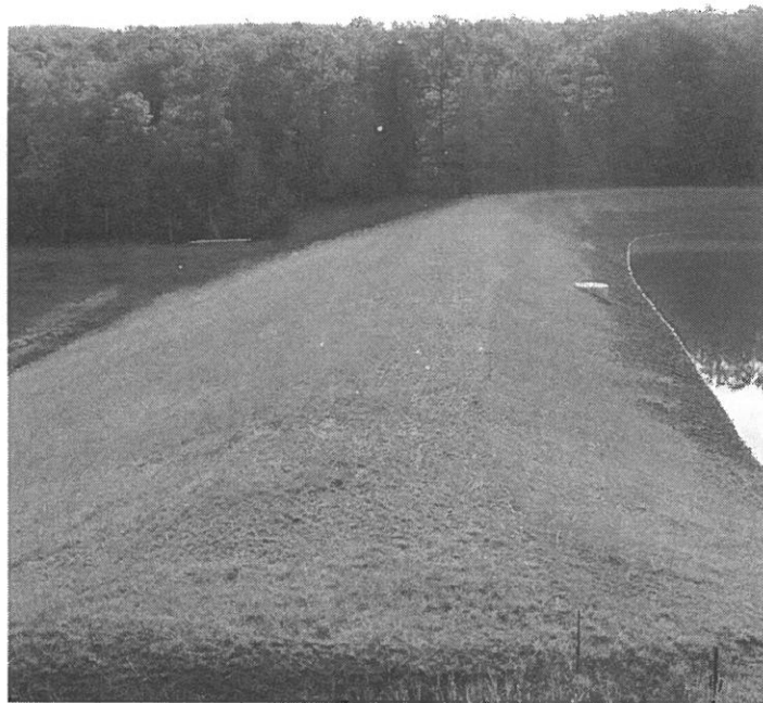
WILSON DAM MODIFICATION, HAMPSHIRE CO., WV
