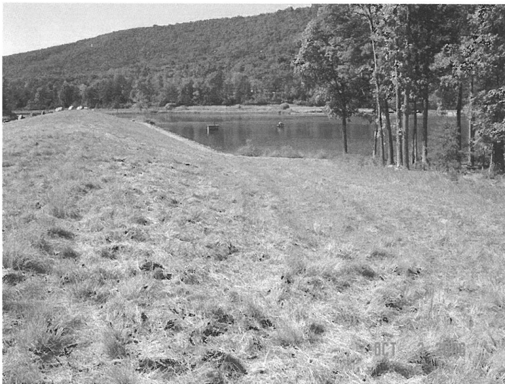
WARDEN LAKE DAM MODIFICATION, HARDY CO., WV
