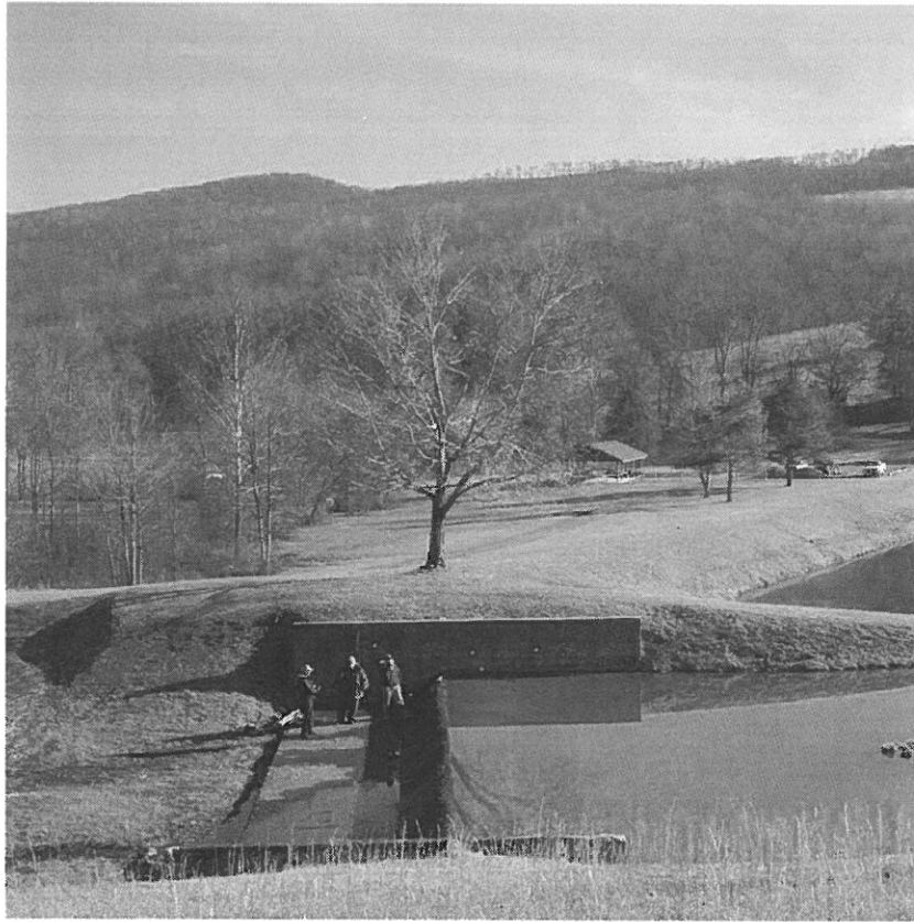
BELINGTON DAM MODIFICATION, BELINGTON, WV
