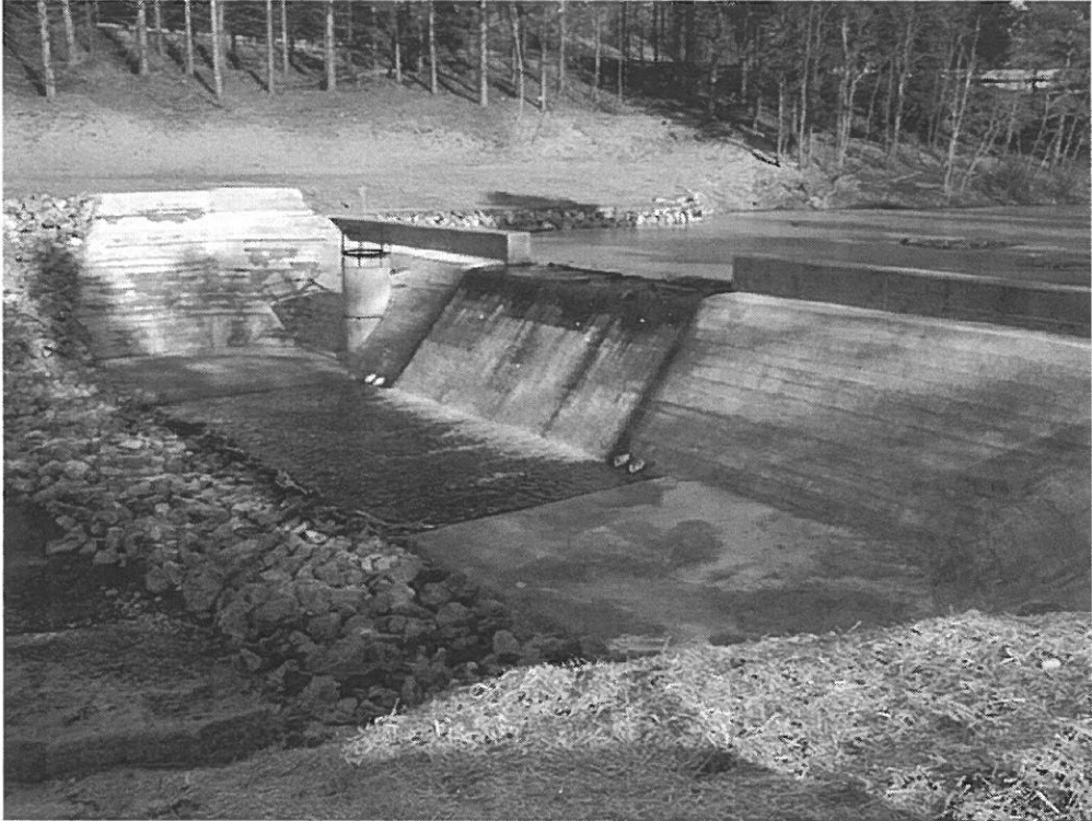
THOMAS DAM MODIFICATION, THOMAS, WV
