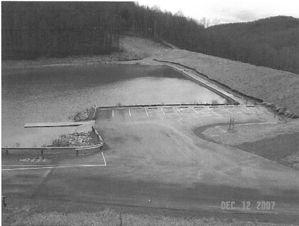
BAILEY DAM MODIFICATION, MONONGALIA CO., WV
