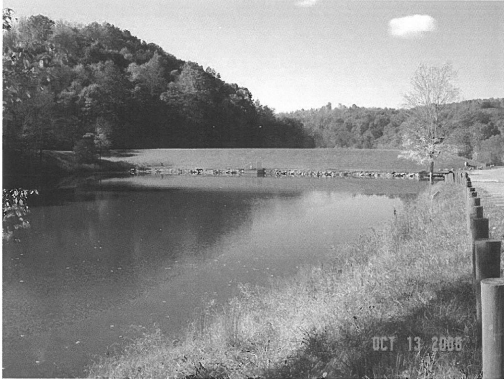
JIMMY LEWIS DAM MODIFICATION, MERCER CO., WV
