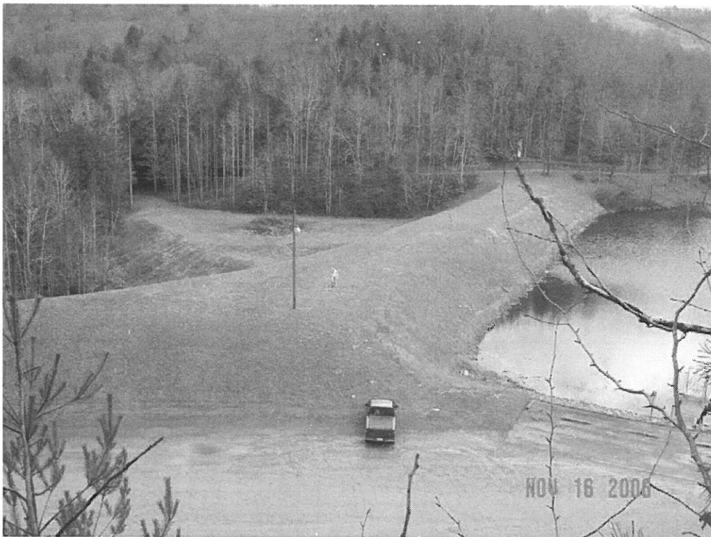
PLUM ORCHARD DAM MODIFICATION, FAYETTE CO., WV
