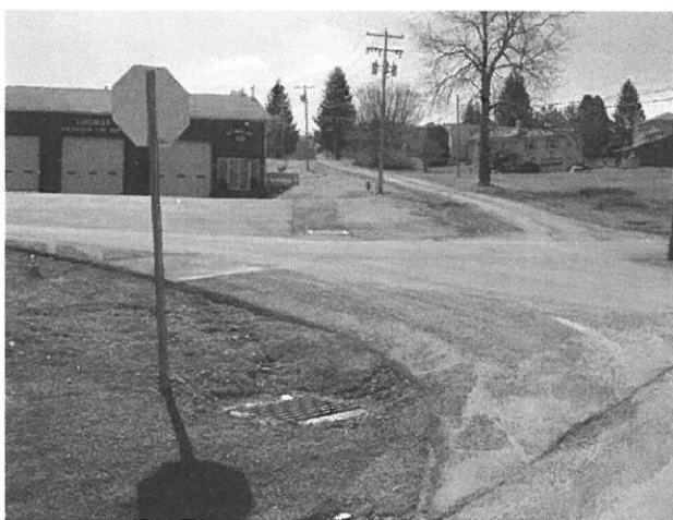
New Storm Drains and Catch Basins
