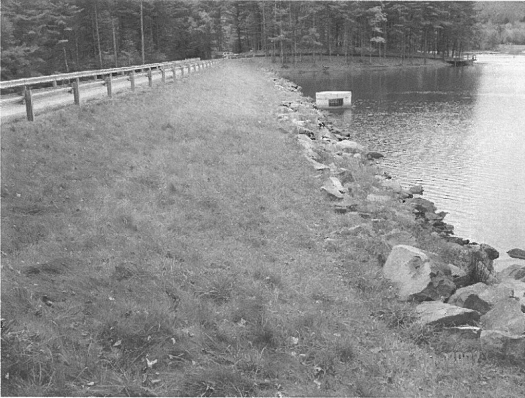
MONCOVE DAM MODIFICATION, MONROE CO., WV
