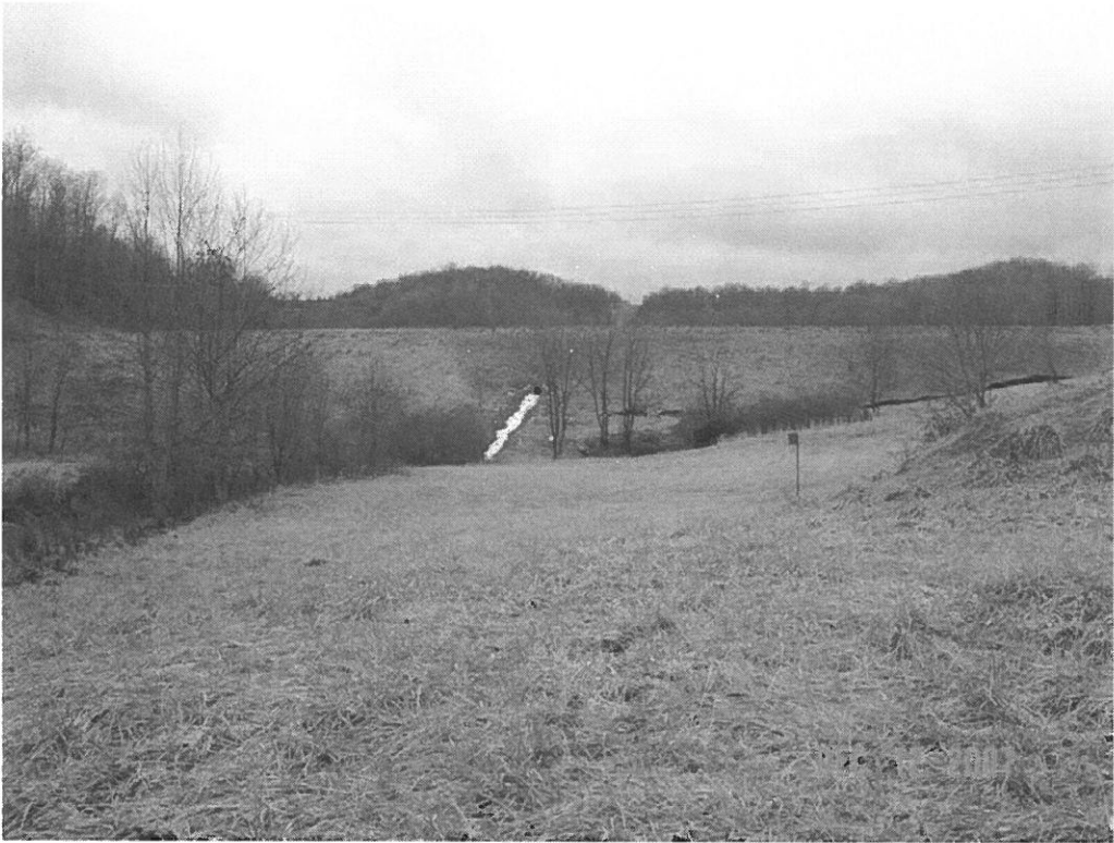
LEMLEY DAM MODIFICATION, MONONGALIA CO., WV
