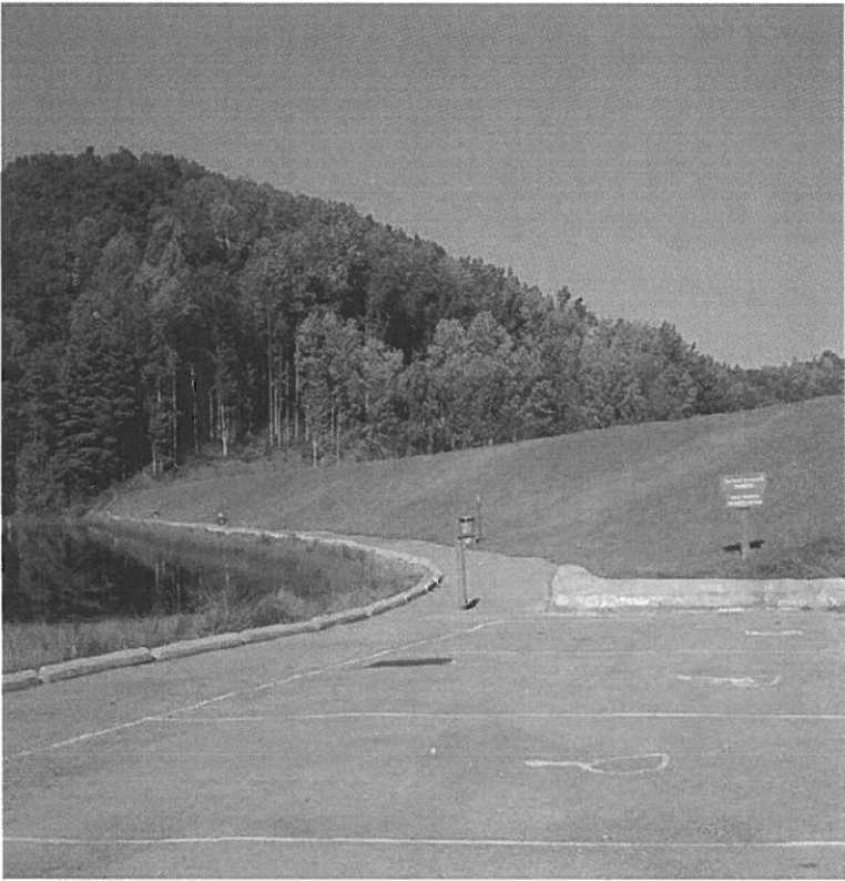
TETER CREEK DAM MODIFICATION, BARBOUR CO., WV
