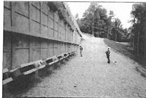
Finished wall with anchors
