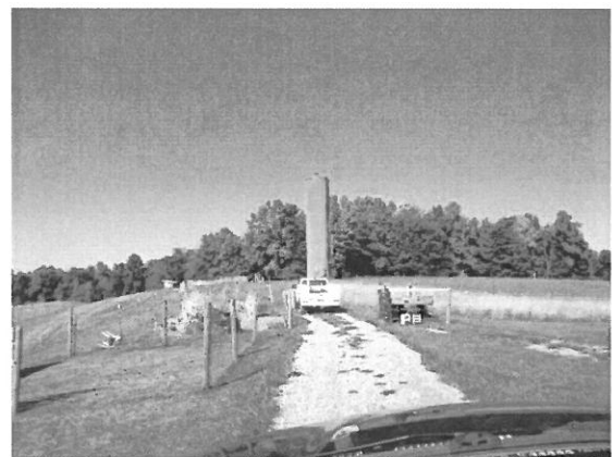
Figure 1: Tank Monitoring Site Extreme Endeavors Controls with the INSCADA System
