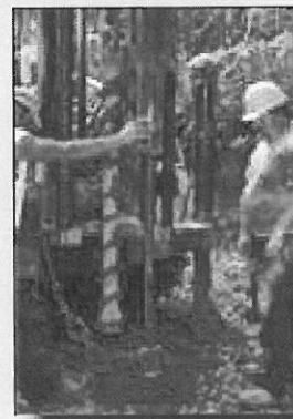
Drilling in Rugged Terrain
