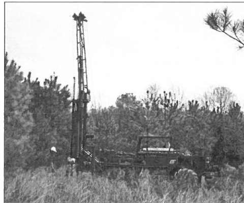
CTL's ATV can drill in rough terrain
