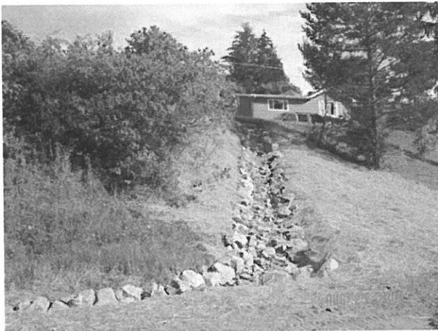
Erosion Repair – Rip Rap Armored Ditch
