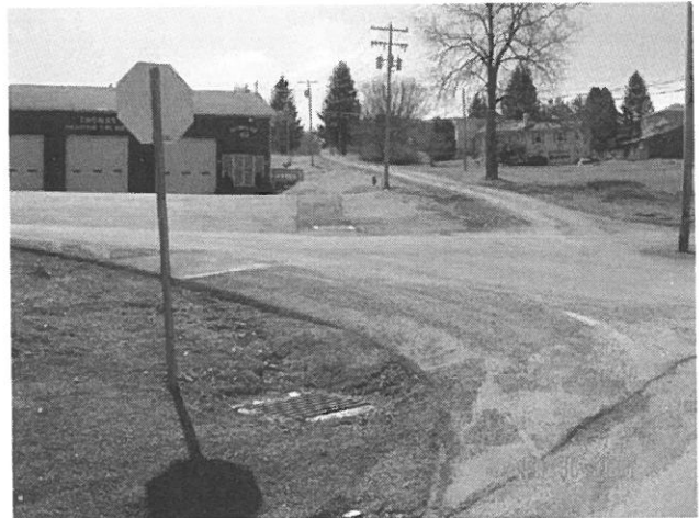
New Storm Drains and Catch Basins
