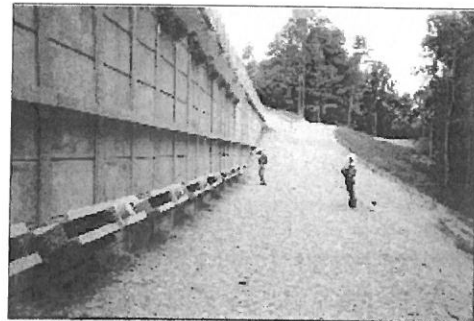
Finished wall with anchors
