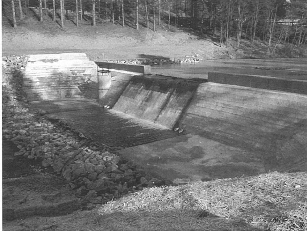
THOMAS DAM MODIFICATION, THOMAS, WV
