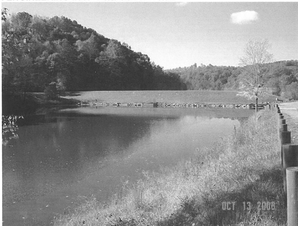
JIMMY LEWIS DAM MODIFICATION, MERCER CO., WV
