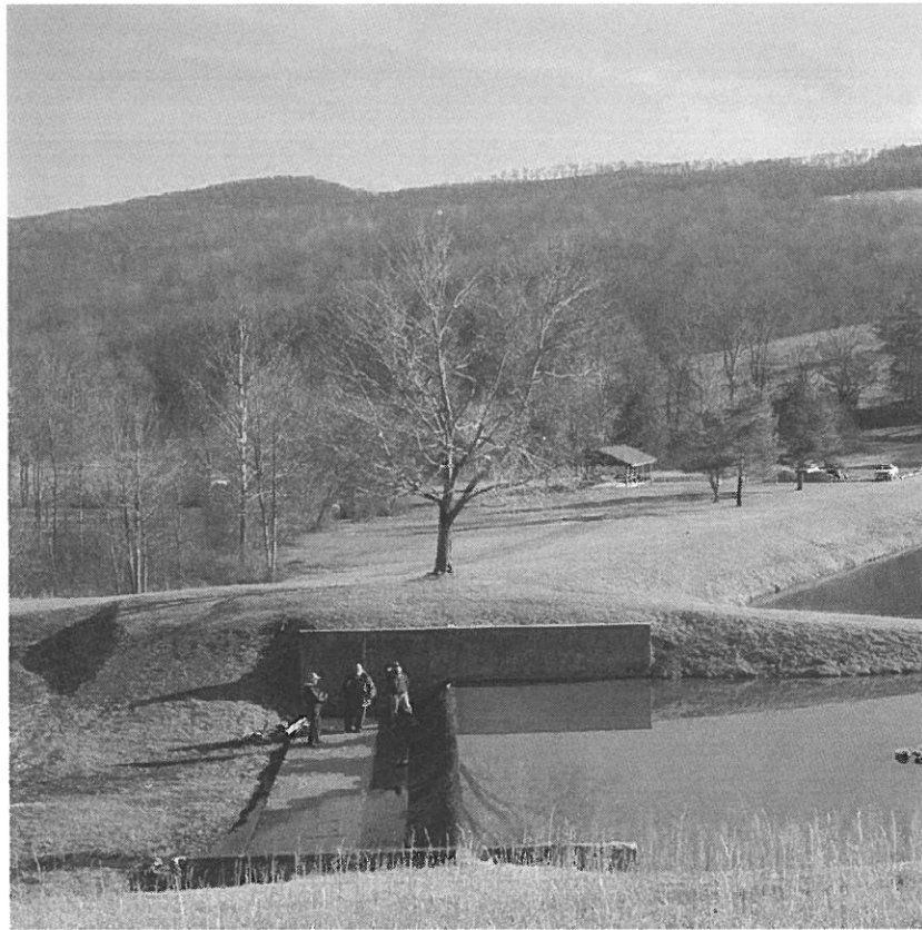
BELINGTON DAM MODIFICATION, BELINGTON, WV
