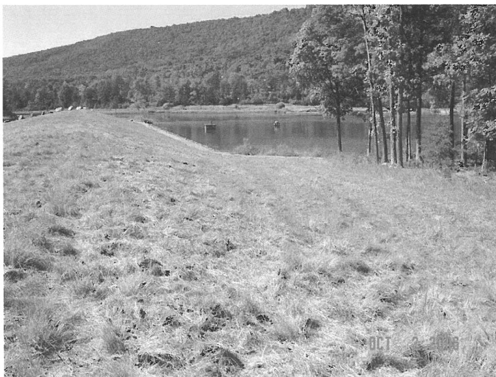
WARDEN LAKE DAM MODIFICATION, HARDY CO., WV
