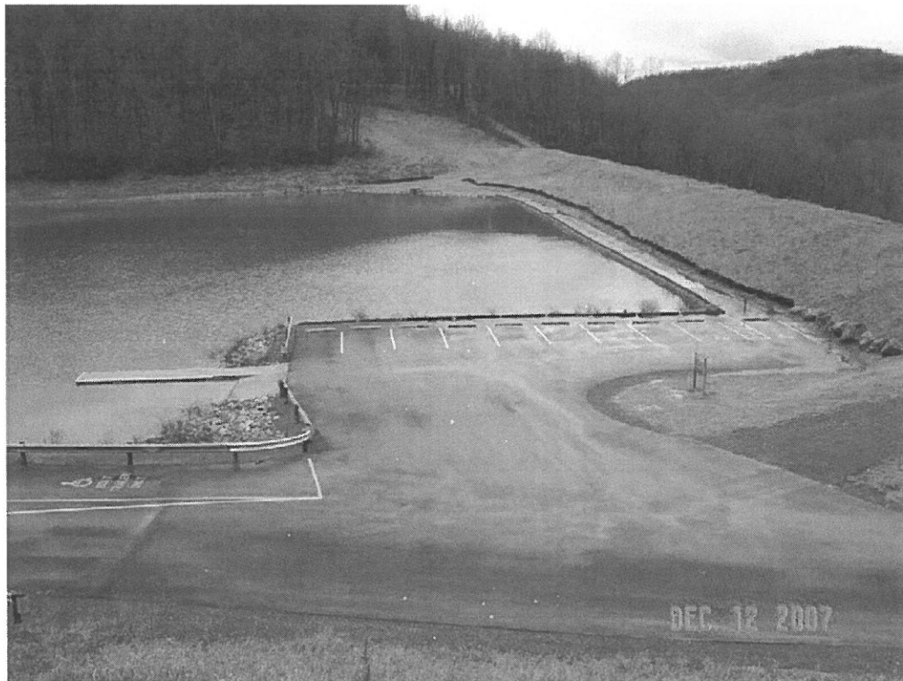
BAILEY DAM MODIFICATION, MONONGALIA CO., WV
