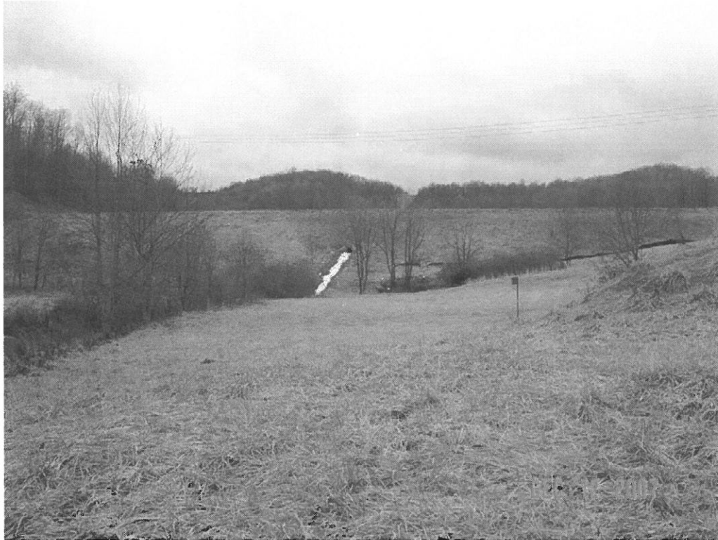
LEMLEY DAM MODIFICATION, MONONGALIA CO., WV
