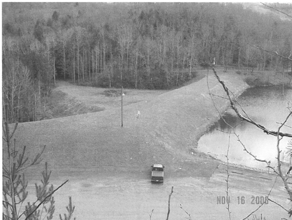
PLUM ORCHARD DAM MODIFICATION, FAYETTE CO., WV
