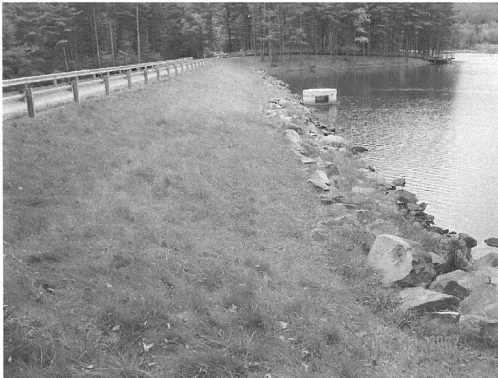
MONCOVE DAM MODIFICATION, MONROE CO., WV
