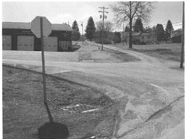
New Storm Drains and Catch Basins
