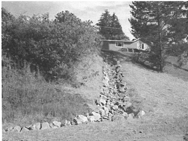
Erosion Repair – Rip Rap Armored Ditch
