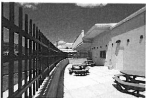
Corbin Utilities Office and Warehouse Buildings, Corbin, KY
