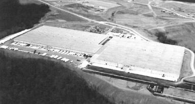
a precast concrete wall panel system was designed for the building shell, and erected onto steel framing. Security lighting was designed for these areas, with careful attention paid to illumination levels to permit camera operation in the parking lot areas.
