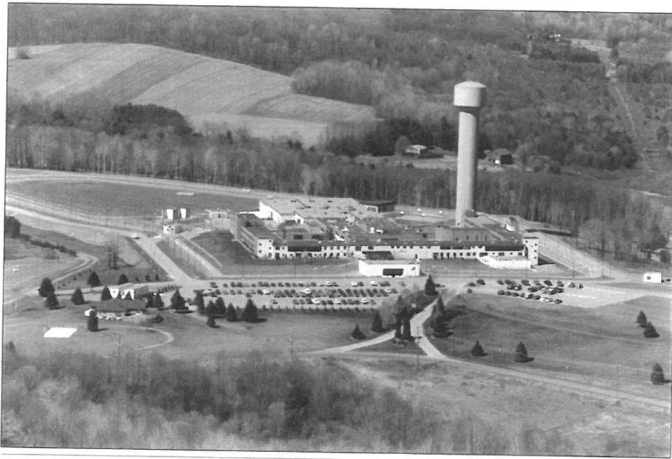
Federal Correctional Institution. The $4.3 million project for the Federal Bureau of Prisons was completed in 1990.
