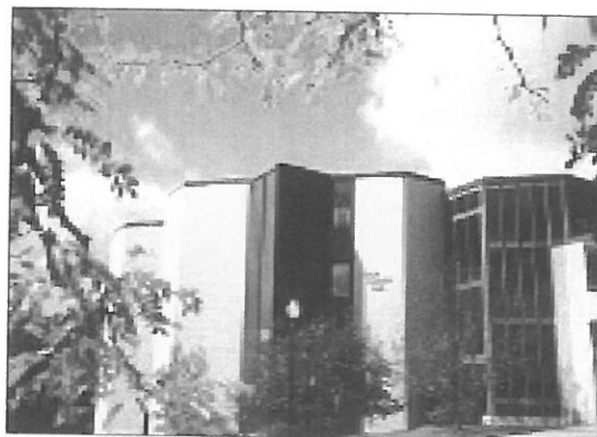
Fairmont State College. H.F. Lenz Company upgraded the electrical distribution system for Hunt Haught Hall.
