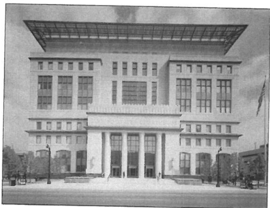
Robert C. Byrd Courthouse. Selected mechanical system commissioning activities were performed for this new seven-story, 325,000 sq.ft. courthouse.
