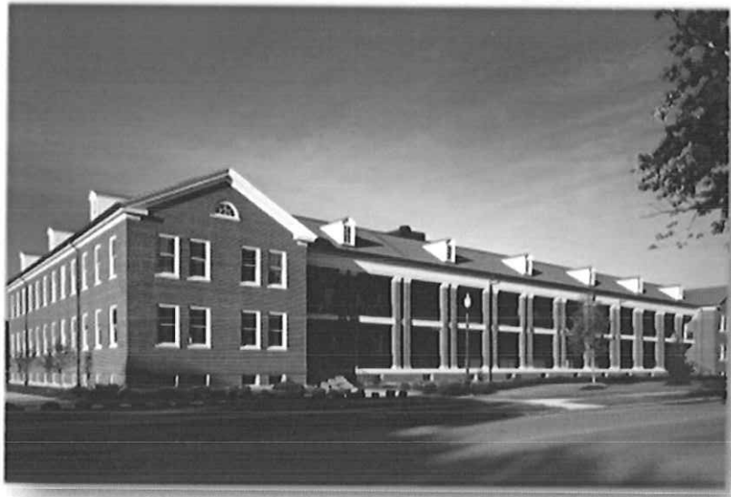
The Schneider Corporation Headquarters at Historic Fort Harrison
