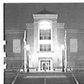
Putnam County Courthouse & Judicial Center -New Judicial Center -Courthouse Addition & Renovation
