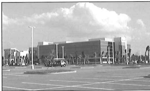
Confidential Insurance Company. The new South-Eastern United States call center building includes employee amenities such as food service, meeting rooms, and training facilities.
