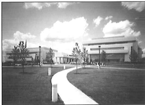
FedEx Ground. The new corporate headquarters contains a raised-floor computer area, an auditorium, a cafeteria, a media production studio, and a fitness center.
