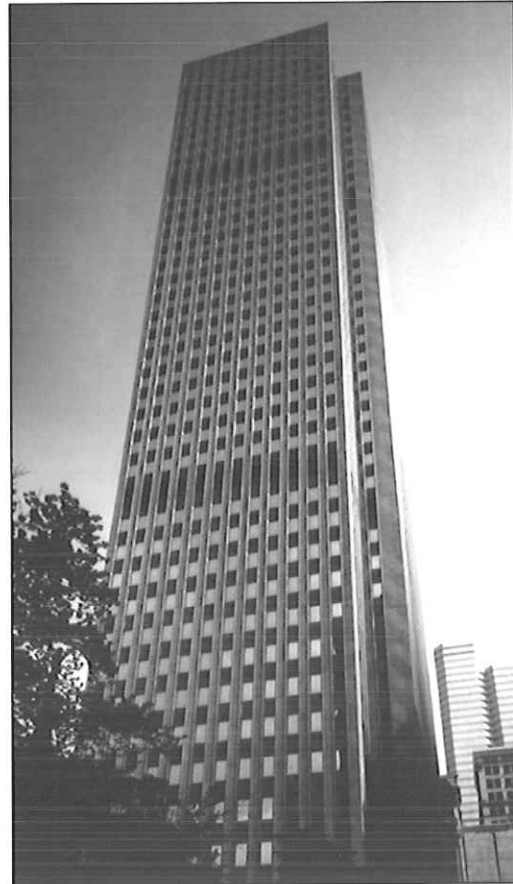
Three Mellon Center. This high-rise was retrofit in the mid-1980's and is currently undergoing a phased modernization program to provide an increased level of reliability for computer operations.
