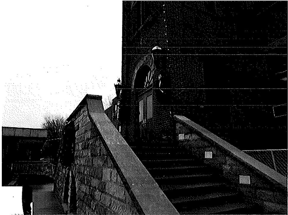
PWWG's scope of work included stripping and repointing all exterior masonry. Main entry before (left) and after (top)
