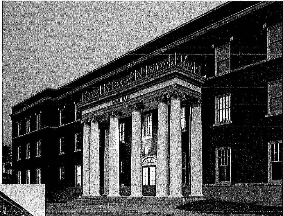
Restored columns and terra cotta entablature at main entry portico (above). Overall view of restored exterior (left).
