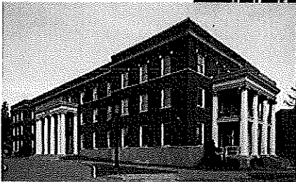
Restored columns and terra cotta entablature at main entry portico (above). Overall view of restored exterior (left).
