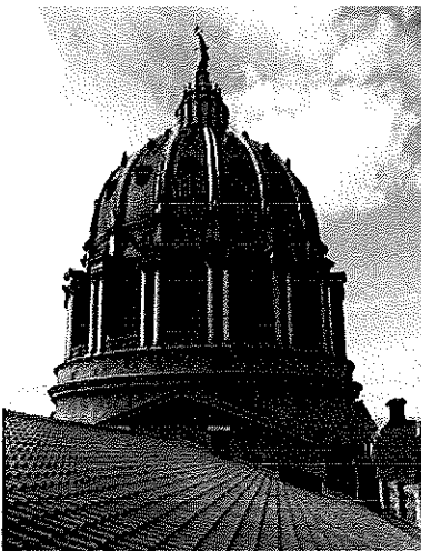
PWWG completed rehab and roof restoration at the PA State Capitol in Harrisburg.
