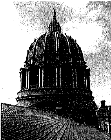
PA Capitol roof and peristyle deck.
