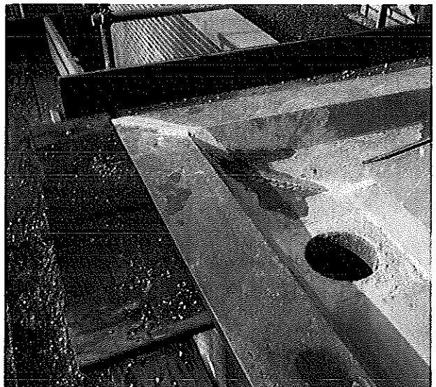
New flashing, coping, and copper gutter to channel rainwater collected from the building's various roofing systems.
