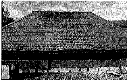
Original slate roof (left) and repair/replacement in progress (right).
