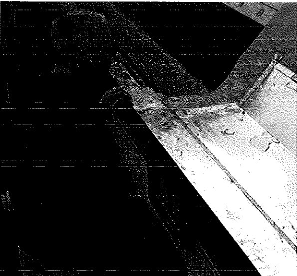
New copper drainage basin and roof drain under construction (left), and near completion (right)
