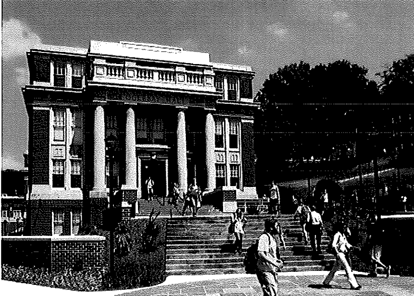
The renovation of Oglebay Hall at WVU Morgantown included installing a new roof on this Historic Register building.
