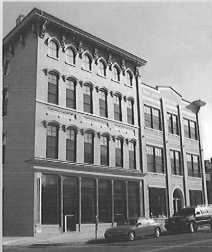
CATHOLIC HERITAGE CENTER Wheeling, West Virginia
