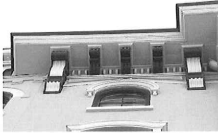
CATHOLIC HERITAGE CENTER Wheeling, West Virginia
