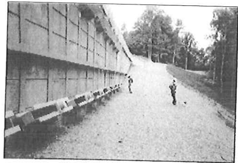
Finished wall with anchors
