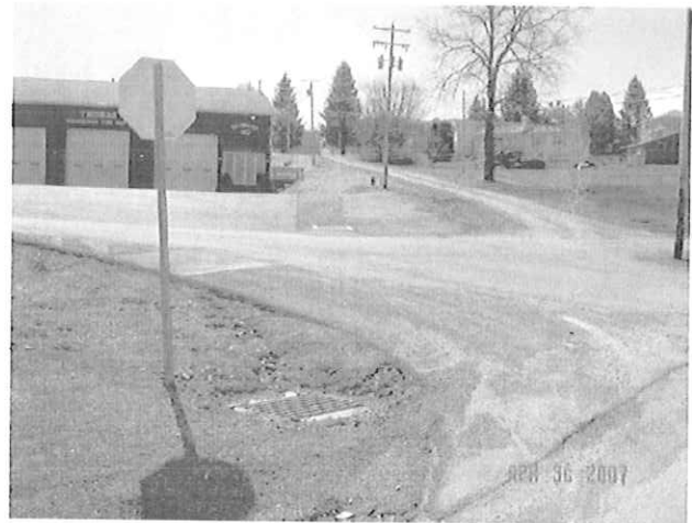
New Storm Drains and Catch Basins
