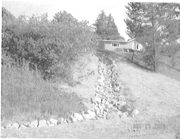
Erosion Repair – Rip Rap Armored Ditch
