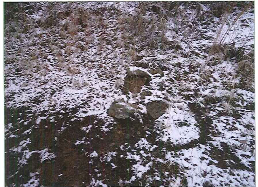
Photo "B" – Seep located below Landslide
