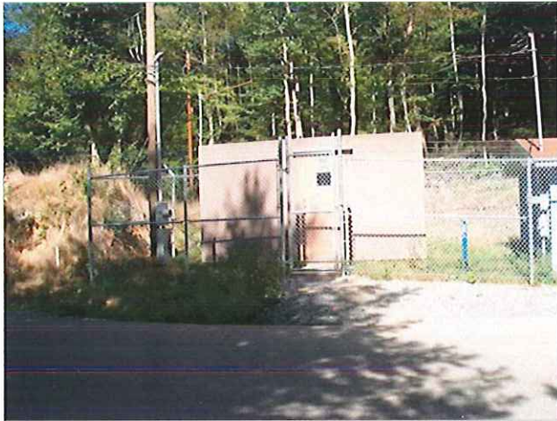
150 GPM Little Sand Run Booster Station
