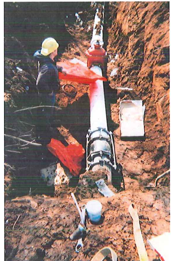
Connection of 10" HDPE River Crossing Pipe (Directionally Drilled) to 10" C-900 Pipe at Tygart Valley River
