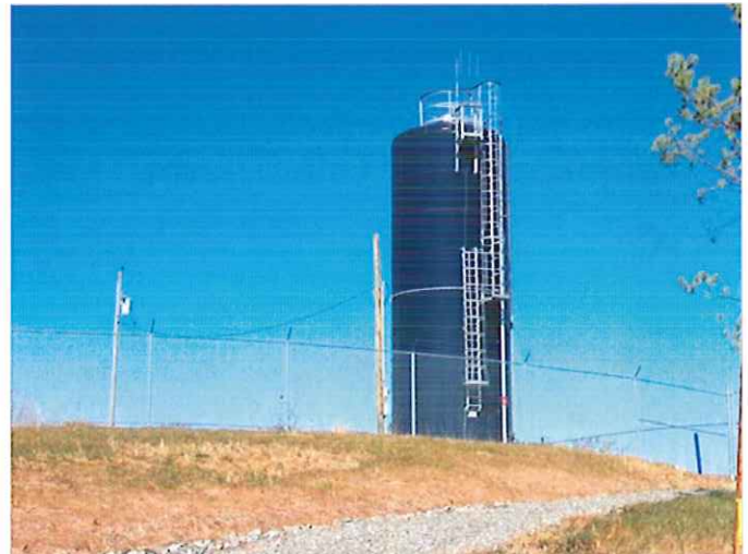
43,000 Gallon Salem Ridge Water Storage Tank
