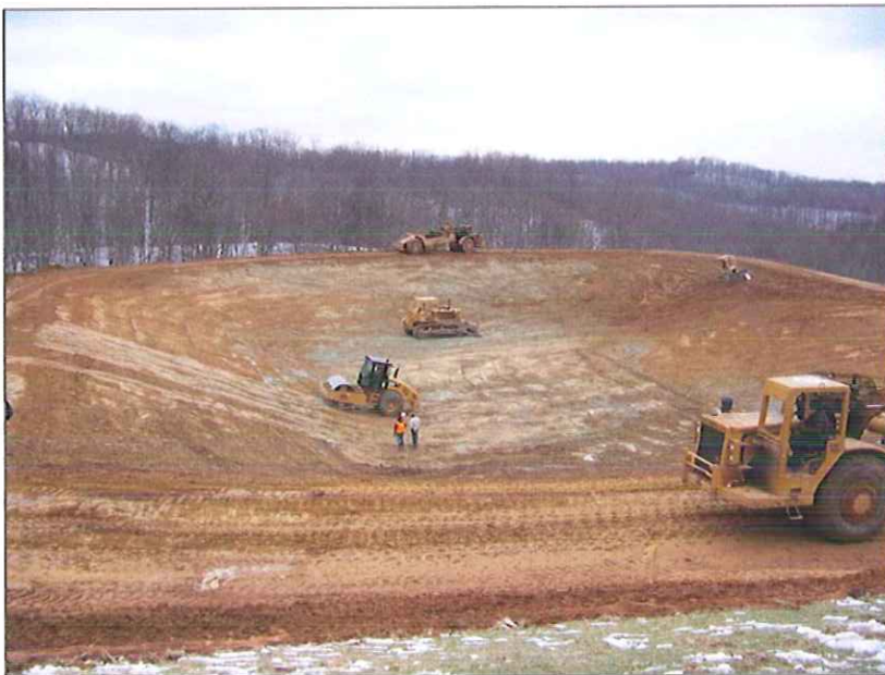
Frac pit site preparation, Ritchie County, WV
