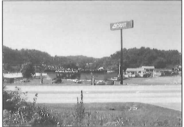
CTL Engineering of West Virginia, Inc. provided site plans for this Advance Auto Parts Store in Morgantown, West Virginia
