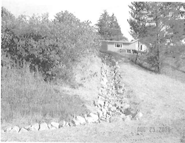
Erosion Repair – Rip Rap Armored Ditch
