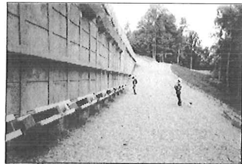
Finished wall with anchors
