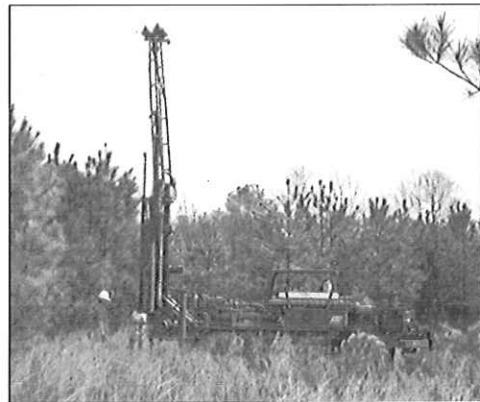
CTL's ATV can drill in rough terrain
