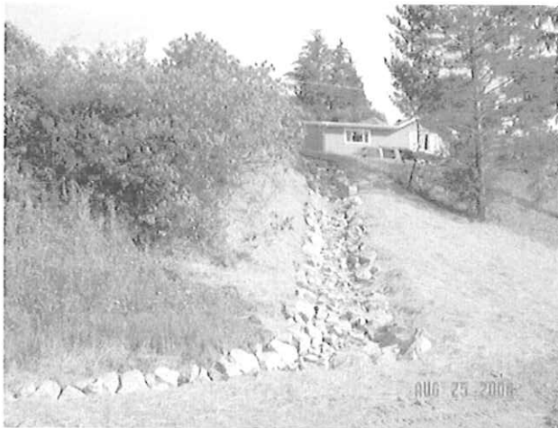
Erosion Repair – Rip Rap Armored Ditch
