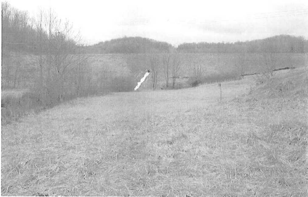
LEMLEY DAM MODIFICATION, MONONGALIA CO., WV
