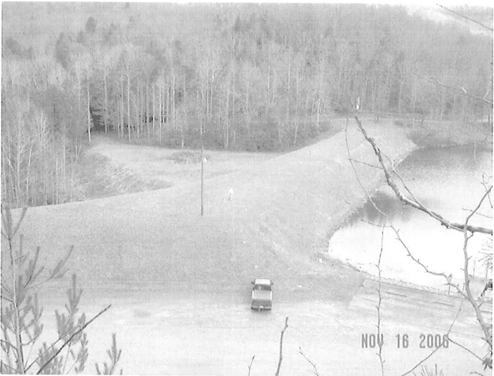
PLUM ORCHARD DAM MODIFICATION, FAYETTE CO., WV
