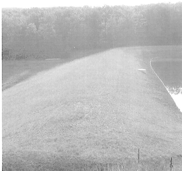
WILSON DAM MODIFICATION, HAMPSHIRE CO., WV
