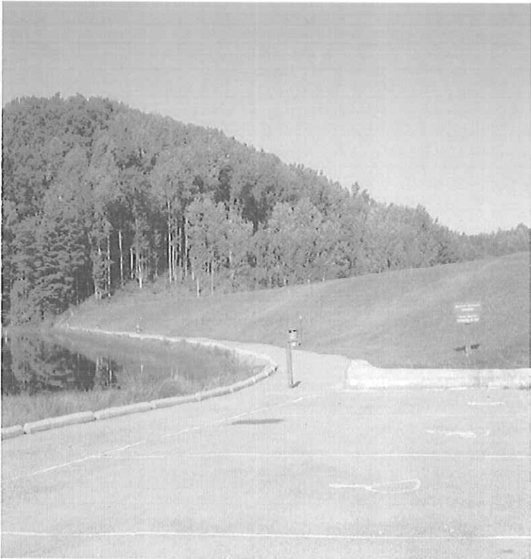
TETER CREEK DAM MODIFICATION, BARBOUR CO., WV
