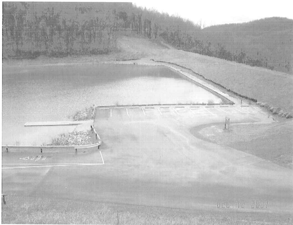
BAILEY DAM MODIFICATION, MONONGALIA CO., WV
