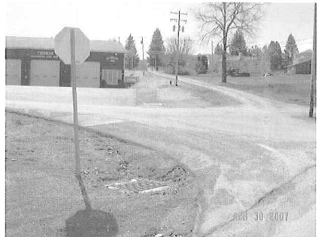
New Storm Drains and Catch Basins
