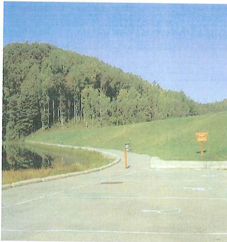
TETER CREEK DAM MODIFICATION, BARBOUR CO., WV
