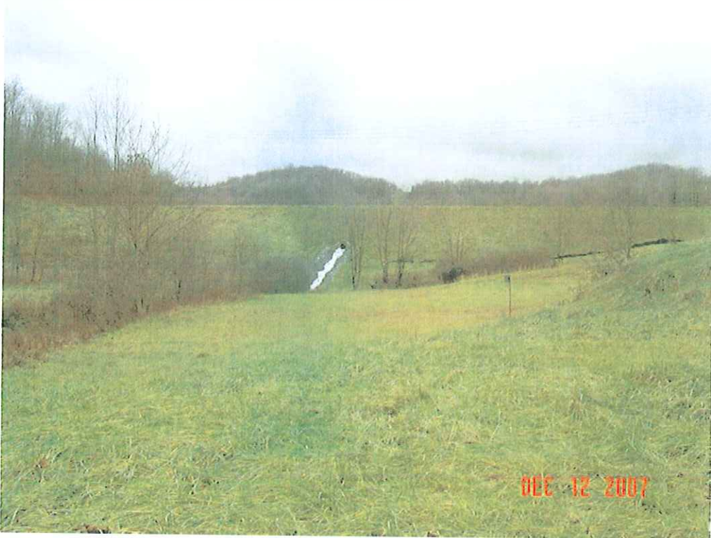
LEMLEY DAM MODIFICATION, MONONGALIA CO., WV
