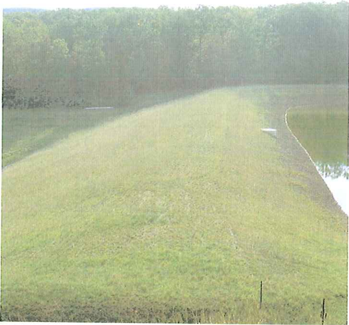
WILSON DAM MODIFICATION, HAMPSHIRE CO., WV
