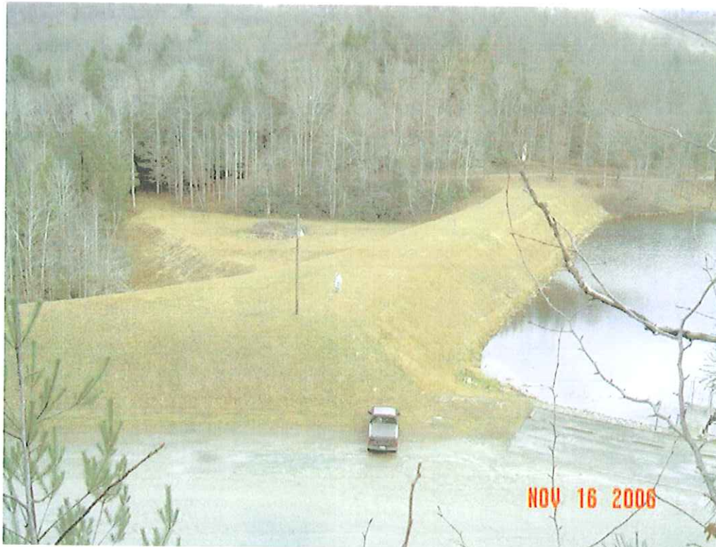
PLUM ORCHARD DAM MODIFICATION, FAYETTE CO., WV
