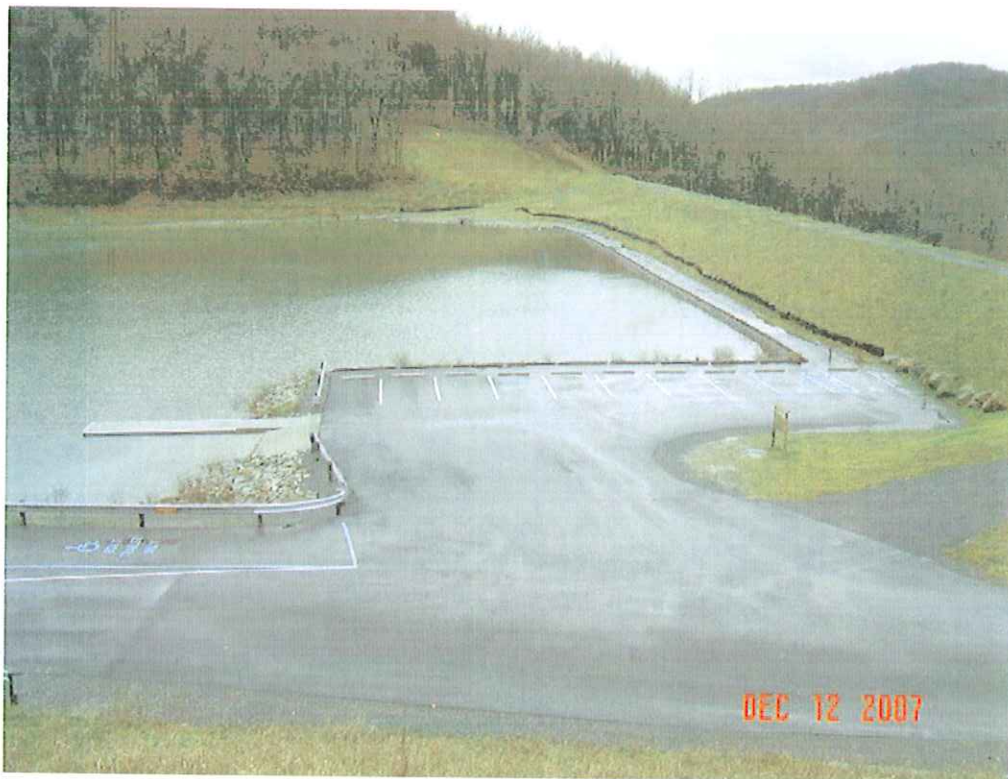
BAILEY DAM MODIFICATION, MONONGALIA CO., WV
