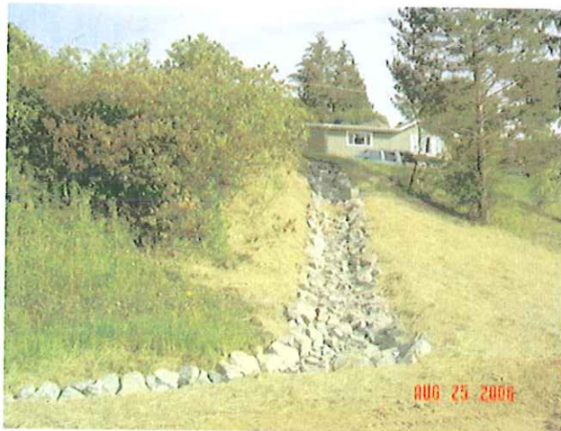
Erosion Repair – Rip Rap Armored Ditch
