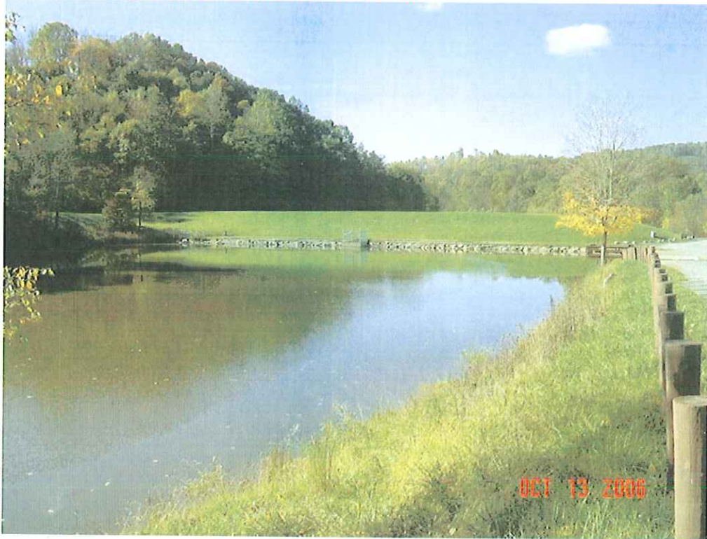
JIMMY LEWIS DAM MODIFICATION, MERCER CO., WV
