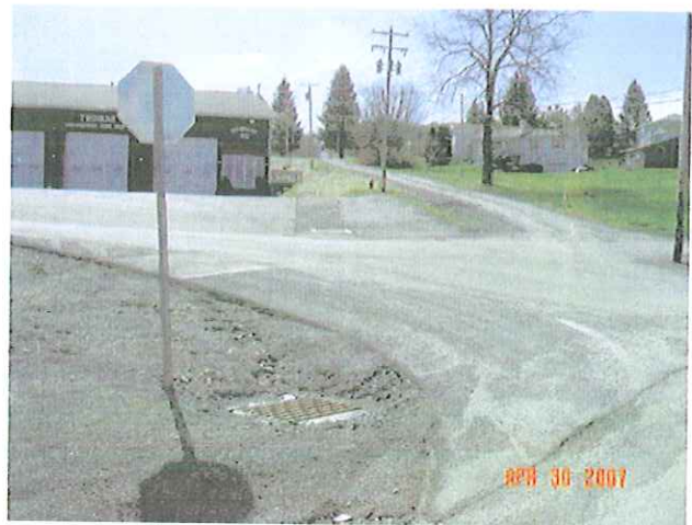
New Storm Drains and Catch Basins
