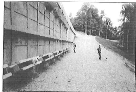
Finished wall with anchors
