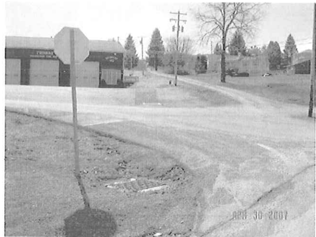
New Storm Drains and Catch Basins
