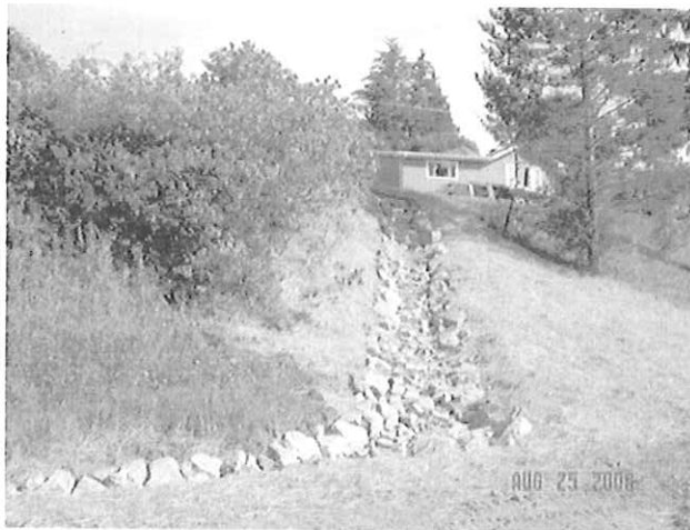
Erosion Repair – Rip Rap Armored Ditch
