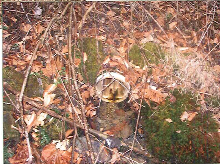
Photo F – Site 5 – Drainage Pipe
