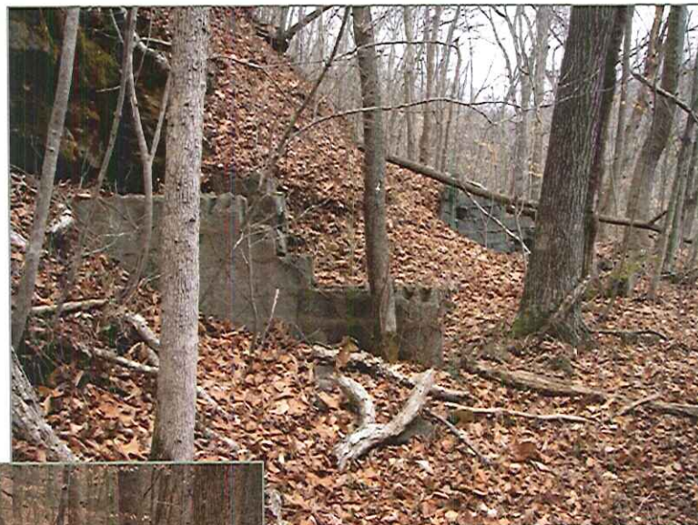
Photo H– Building Foundation
