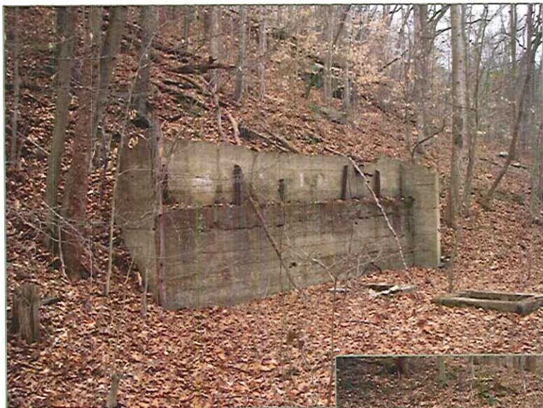
Photo G– Mine Loadout Structure
