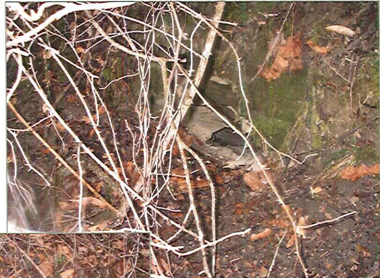
Photo E – Site 5 – Portal
