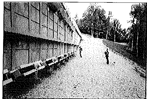
Finished wall with anchors
