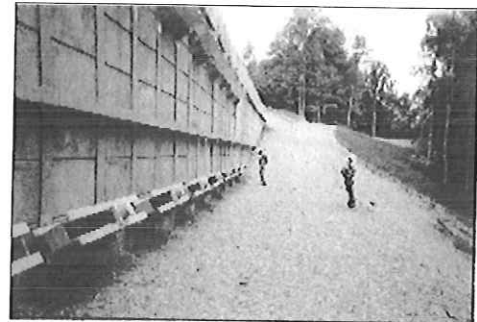
Finished wall with anchors
