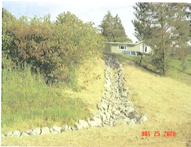
Erosion Repair – Rip Rap Armored Ditch
