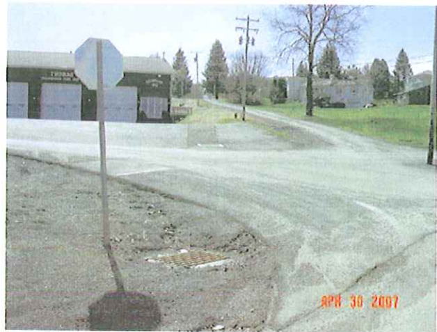
New Storm Drains and Catch Basins
