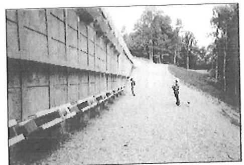
Finished wall with anchors
