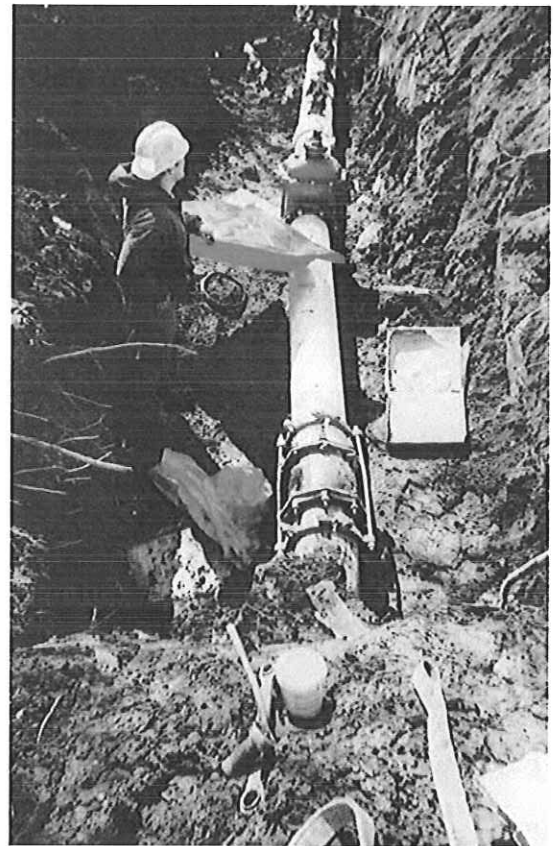
Connection of 10" HDPE River Crossing Pipe (Directionally Drilled) to 10" C-900 Pipe at Tygart Valley River
