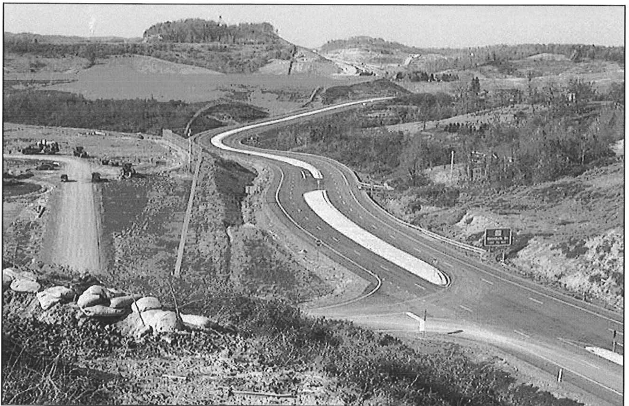
ROUTE 279, NORTH BRIDGEPORT BYPASS – COMPLETED IN 2000
