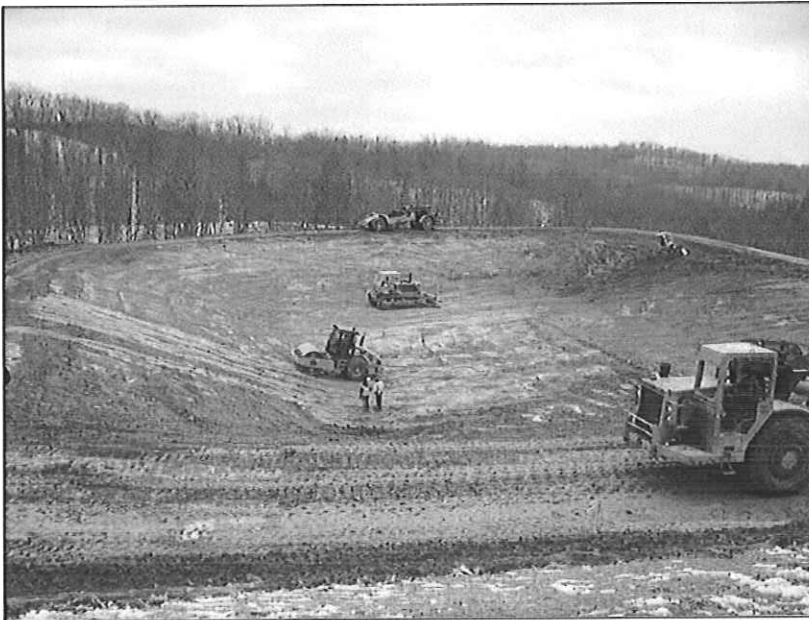
Frac pit site preparation, Ritchie County, WV
