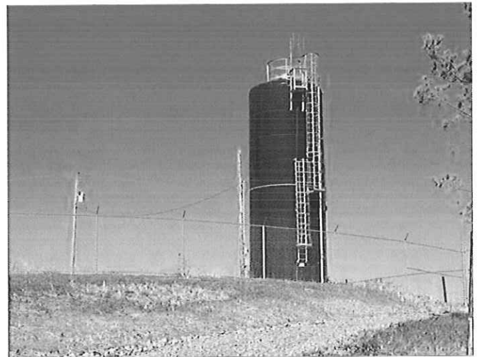
43,000 Gallon Salem Ridge Water Storage Tank
