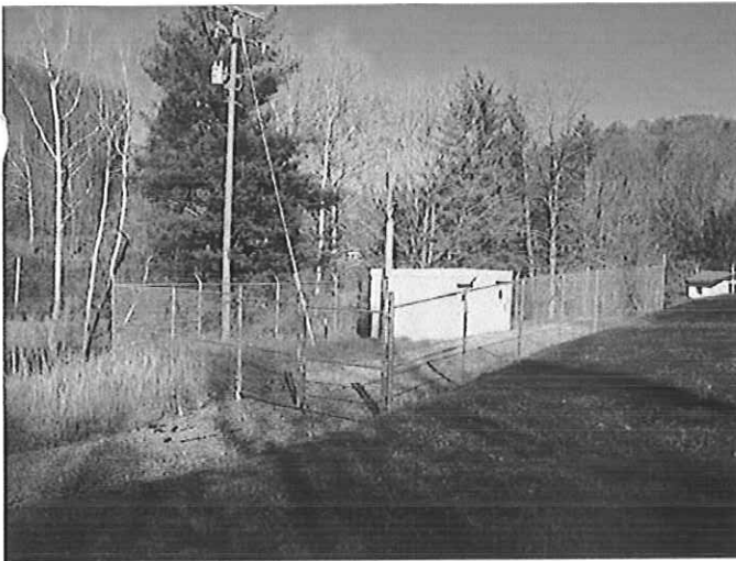
50 GPM Wilsontown Booster Station
