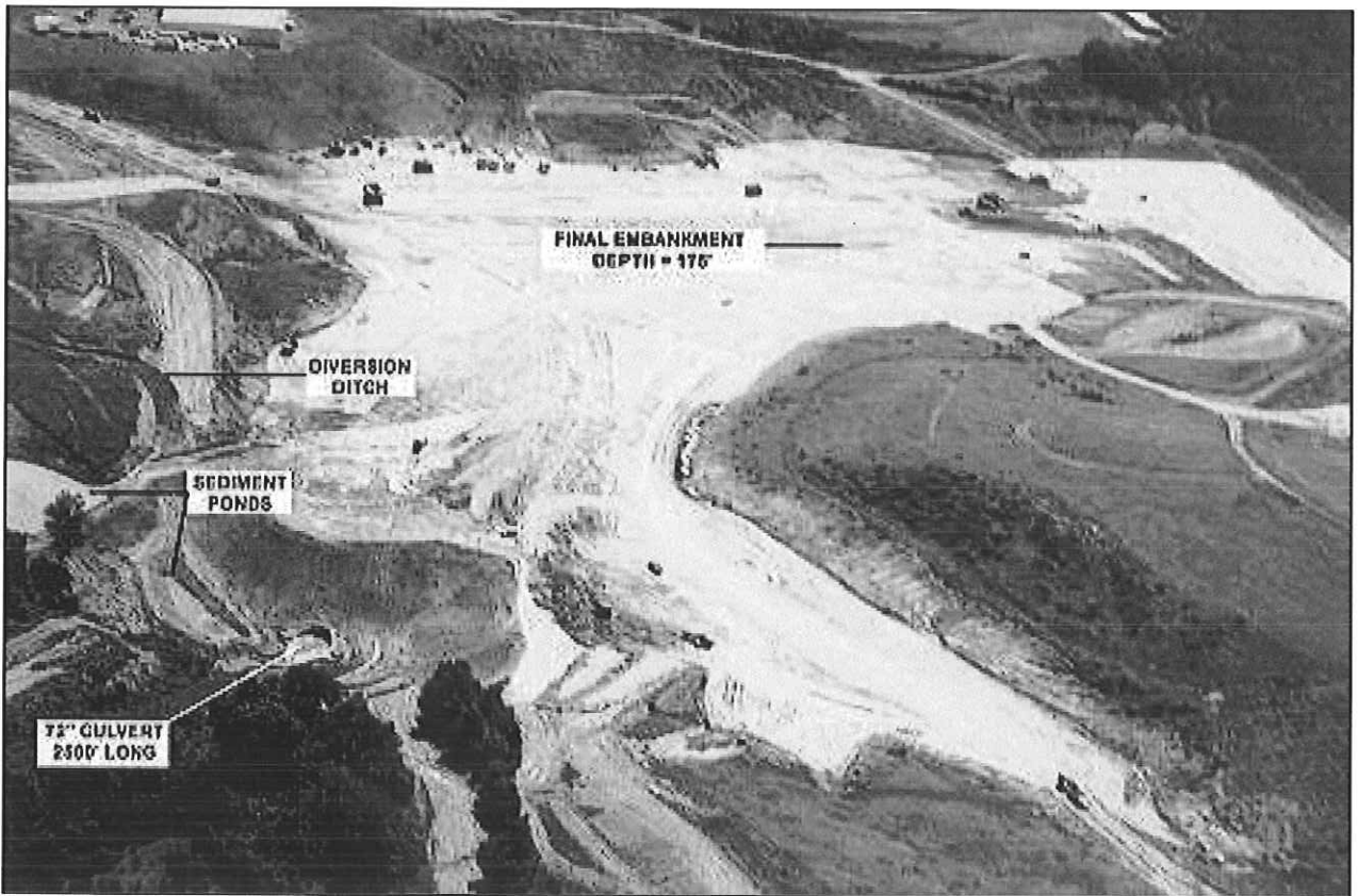
BENEDUM AIRPORT RUNWAY EXTENSION PROJECT - 1999
