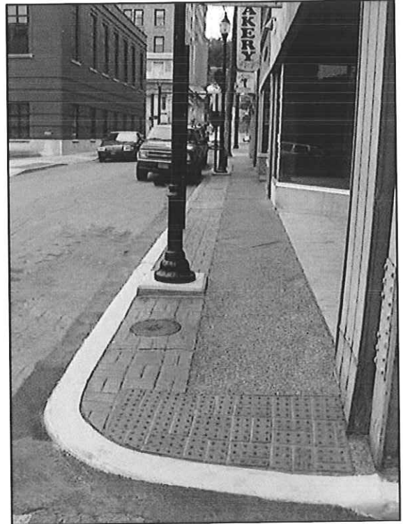
West Side of South Third Street
