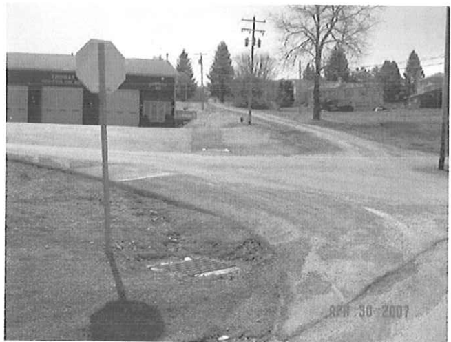
New Storm Drains and Catch Basins
