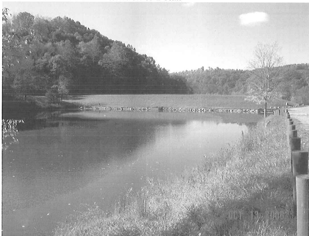
JIMMY LEWIS DAM MODIFICATION, MERCER CO., WV
