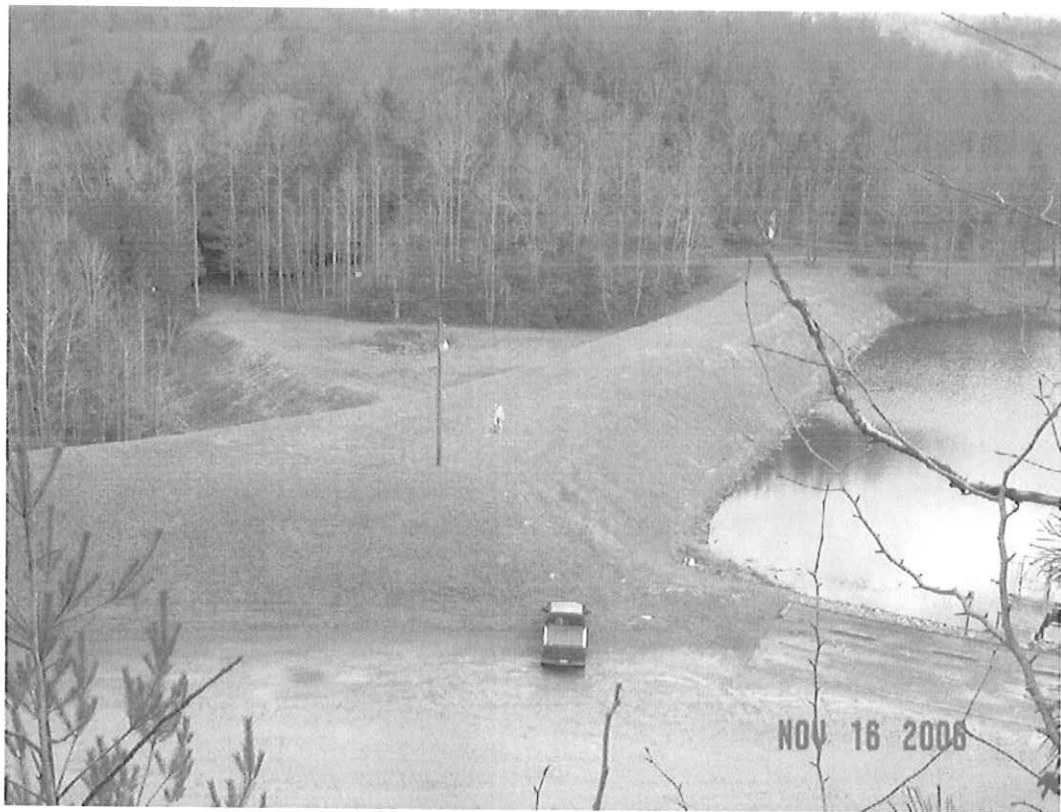
PLUM ORCHARD DAM MODIFICATION, FAYETTE CO., WV
