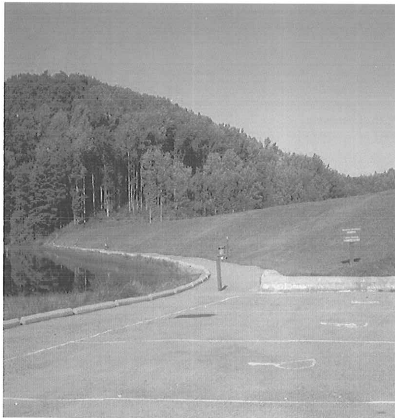
TETER CREEK DAM MODIFICATION, BARBOUR CO., WV
