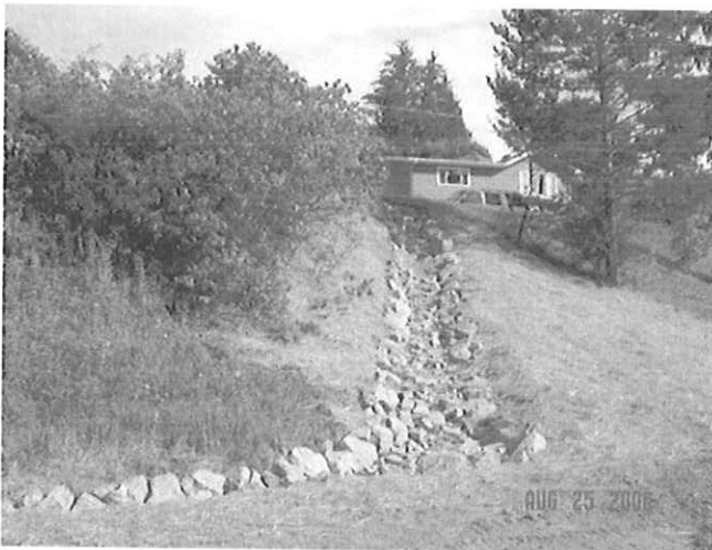
Erosion Repair – Rip Rap Armored Ditch
