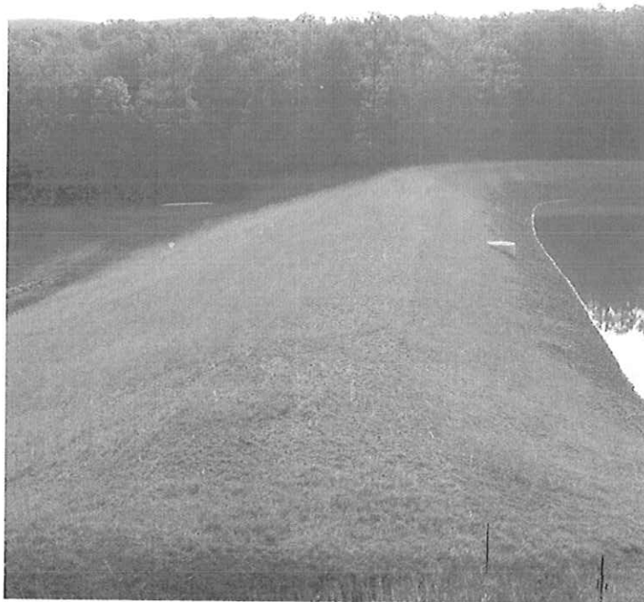
WILSON DAM MODIFICATION, HAMPSHIRE CO., WV
