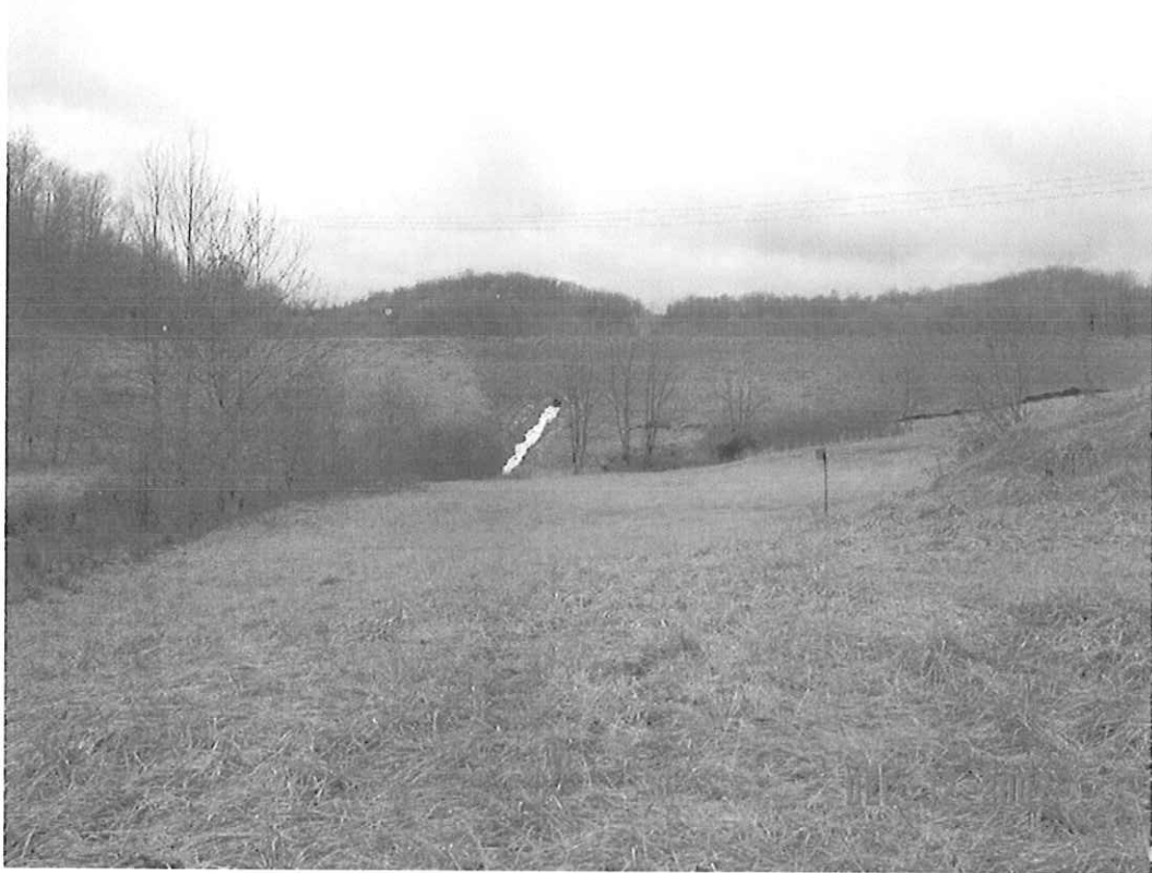
LEMLEY DAM MODIFICATION, MONONGALIA CO., WV
