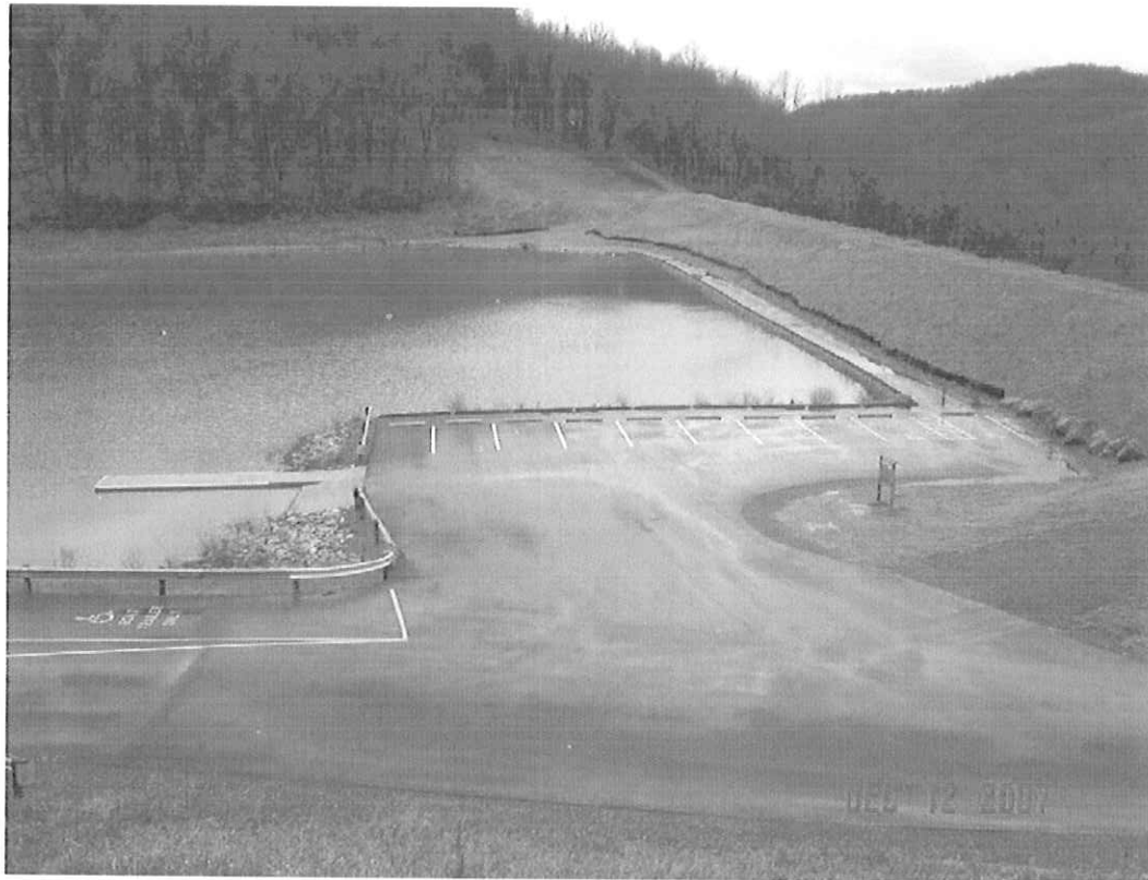
BAILEY DAM MODIFICATION, MONONGALIA CO., WV
