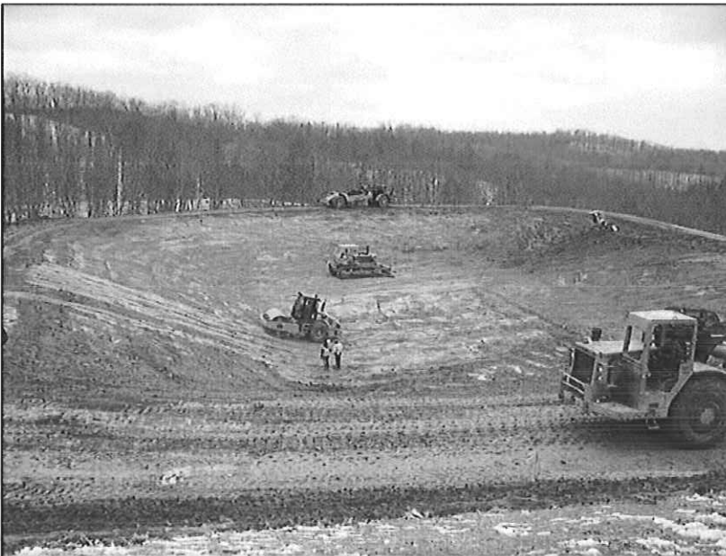
Frac pit site preparation, Ritchie County, WV
