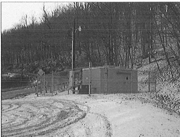
250 GPM Water Booster Station on Route 20
