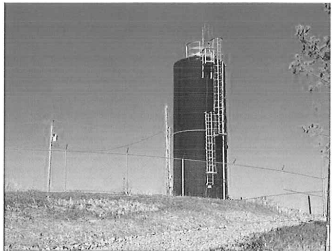
43,000 Gallon Salem Ridge Water Storage Tank
