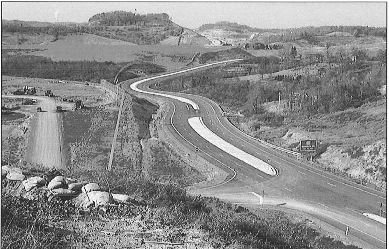
ROUTE 279, NORTH BRIDGEPORT BYPASS – COMPLETED IN 2000
