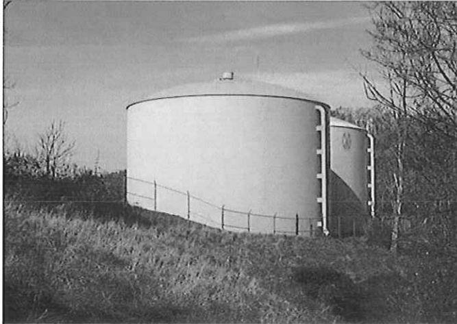
Total Project Cost = $4,400,000 Two 1,000,000 Gallon Storage Tanks Part of FBI Water Project
