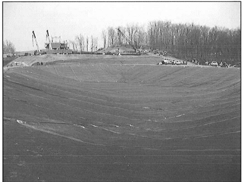
Lined frac pit and drill pad site, Ritchie County, WV
