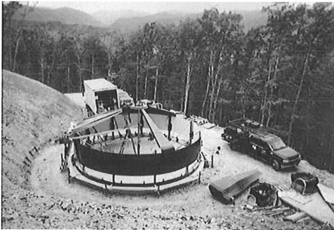
158,000 Gallon Becky's Creek Storage Tank and Site Under Construction
