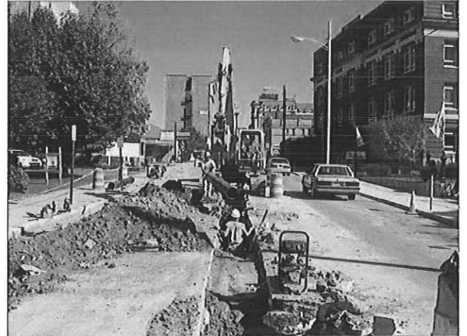
Main Street Waterline Replacement Project New 12" Ductile Iron Pipe Installation
