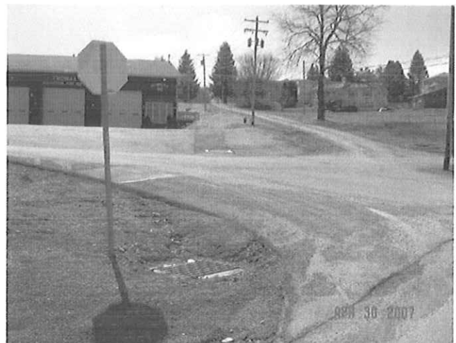
New Storm Drains and Catch Basins
