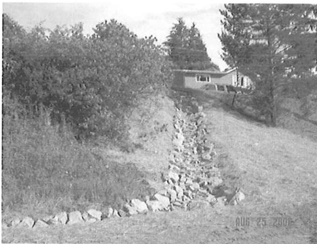
Erosion Repair – Rip Rap Armored Ditch
