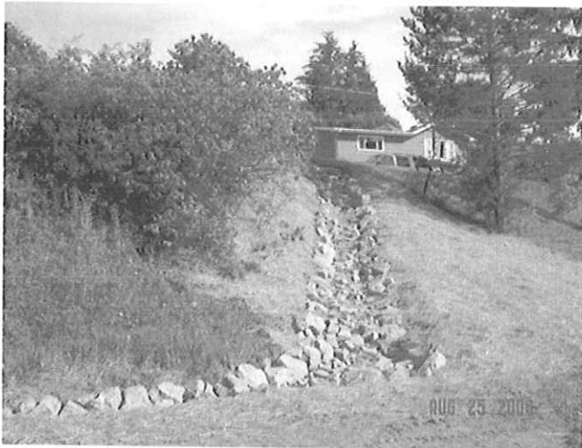
Erosion Repair – Rip Rap Armored Ditch
